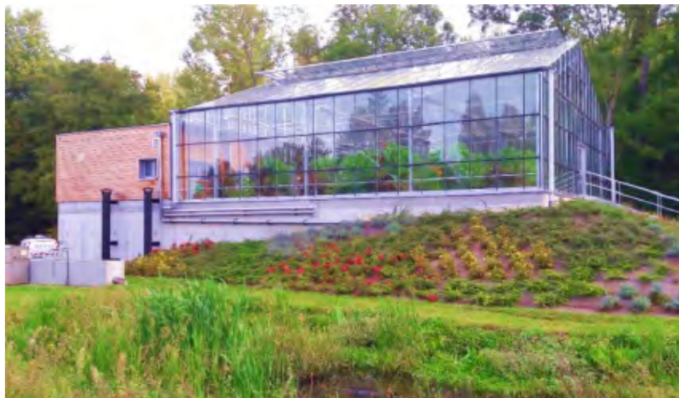
Figure 114 : Station Organica de Nogent-sur-Vernisson (41) - 3 500 EH
